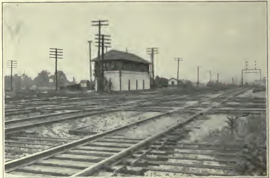
FIG. 259. GRADE CROSSINGS. Crossing of the Illinois Central Railroad with the Pittsburgh, Cincinnati, Chicago & St. Louis Railway and the Baltimore & Ohio Chicago Terminal Railroad, near Riverdale.
